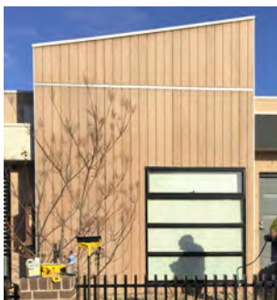
36 MONTHS: The boards are now very light, and are about to begin to be restored.
