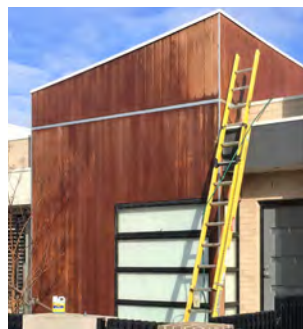
CLEANING: Wash the boards with a deck cleaner and a firm brush.
